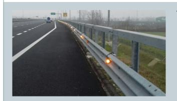
The user support System for foggy weather also provides anti-fog junction delineators, controlled by the fog sensors and supervised by the User Service Centre. The delineators are positioned in correspondence to the acceleration and deceleration lanes of the highway and integrated into the safety barrier.
