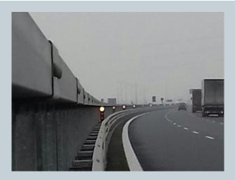
Through a series of fog detection sensors, equipped with high efficiency optical vision, the system perceives the visibility distance, it processes it with humidity data collected and activates, if necessary, the device for foggy weather conditions.
