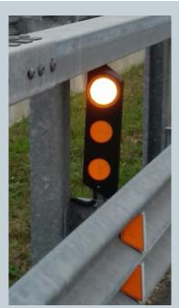
The Fog System consists of LED lighting devices positioned on the safety barriers which delimits the central reservation.
