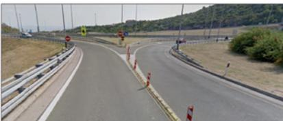
Number of cases with wrong-way driving could be reduced by separating the opposite directions with a physical barrier and an adequate static signalisation. This solution was implemented on the Rijeka bypass junctions. The road marker installation, as shown below (the so-called «snake»), significantly reduced the number of cases where vehicles entered in the wrong direction on the Rijeka bypass.
