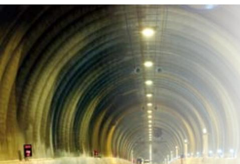
A particular and careful attention is to be paid to the design of tunnels and the respect of high safety standards. These standards are guaranteed both by structural features (e.g. dual-bore tunnel), and by management and emergency systems. Actually, tunnels are equipped with a large number of devices to control and regulate traffic, to communicate with users
